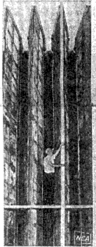
ONE-WAY SOUND TRACK allows air to enter, but keeps jet engine noise from backing out. The acoustical baffles, part of a Koppers noise-suppression system, are at one end of a giant new jet engine test cell in Burbank, Calif., which will be used to test 747s and on-coming breed of supersonic (SST) engines.
